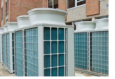
Variable refrigerant flow (VRF) is an HVAC technology that provides energyefficient comfort control for a building's occupants according to the needs of various zones throughout the facility. Supported by integrated controls and sensors, VRF
